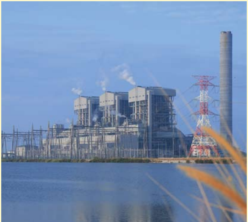
Sultan Azlan Shah Power Station in Perak, Malaysia
